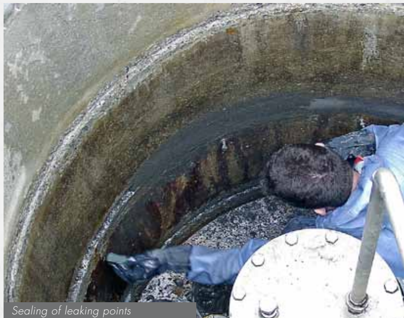
Substrate preparation
