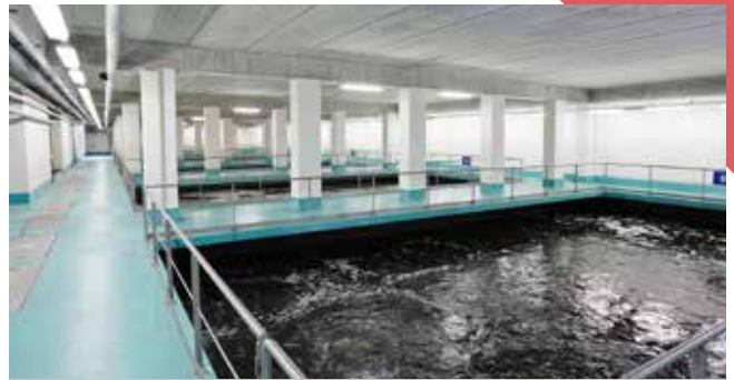
Switzerland: Geneva Sewage Treatment Plant
