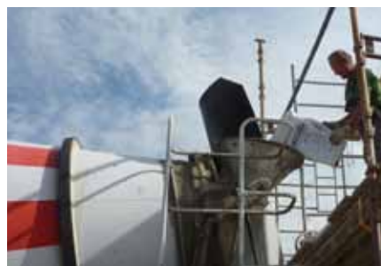
VANDEX AM 10 added at the batching plant.
